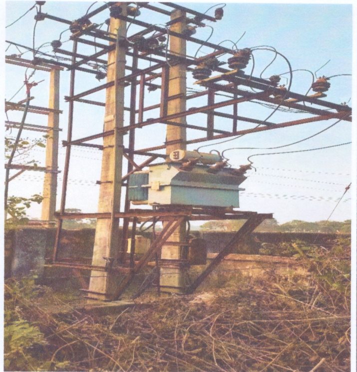
Fig-1 Power supply source Transformer
